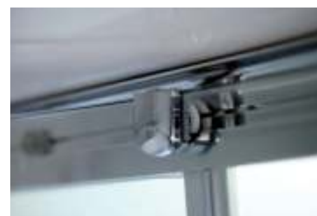
Scorrimento delle ante Sliding door mechanism
